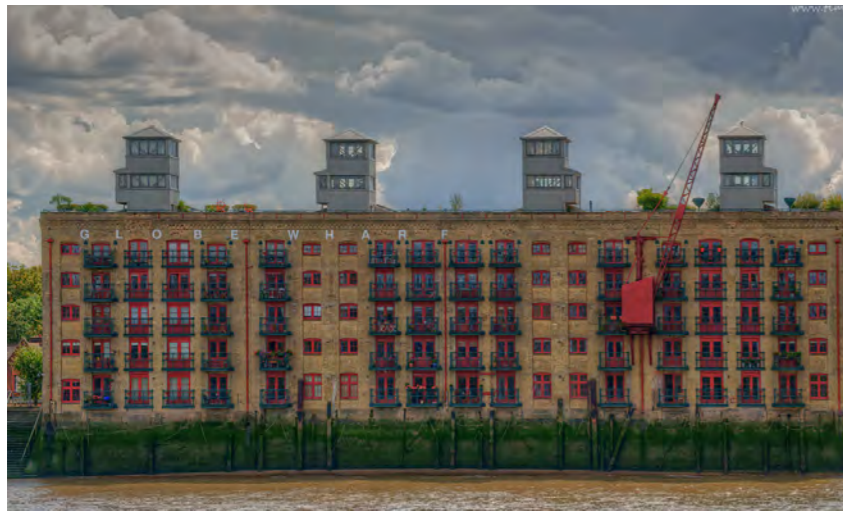
Globe Wharf - adapted former warehouse
