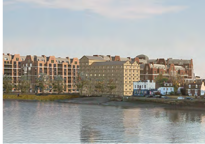
View of The Maltings following reduction in building heights in now Proposed Scheme
