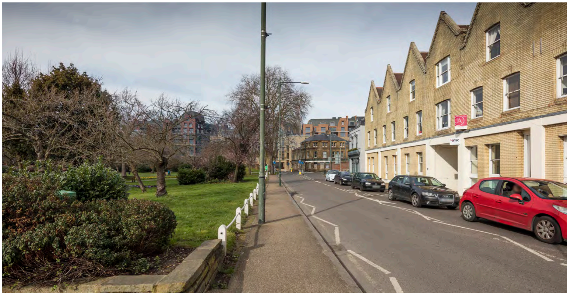
View of the massing of the now Proposed Scheme seen from Sheen Lane by Mortlake Green, showing the proposals massing stepping up gradually in the local context.
