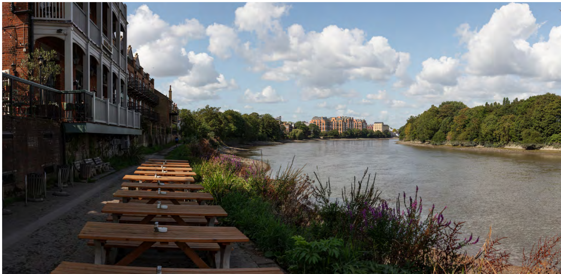
View of the massing of the now Proposed Scheme, indicating it sitting comfortably at the riverfront and set away from The Maltings which retains prominence.
