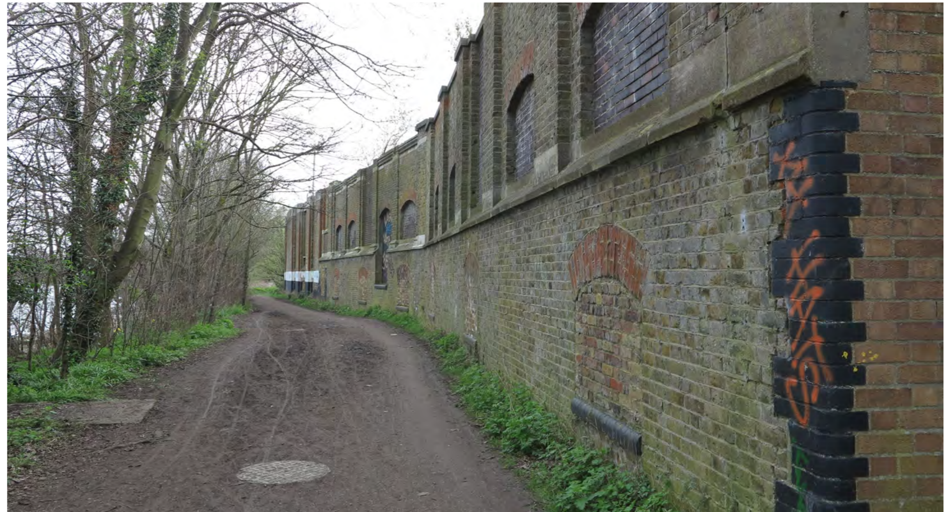
Photograph of existing Northern boundary wall
