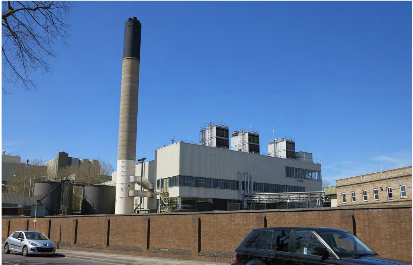
Existing power/ boiler house
