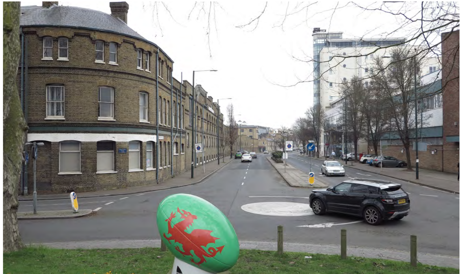
View of existing former hotel and bottling building and Mortlake High Street from Mortlake Green
