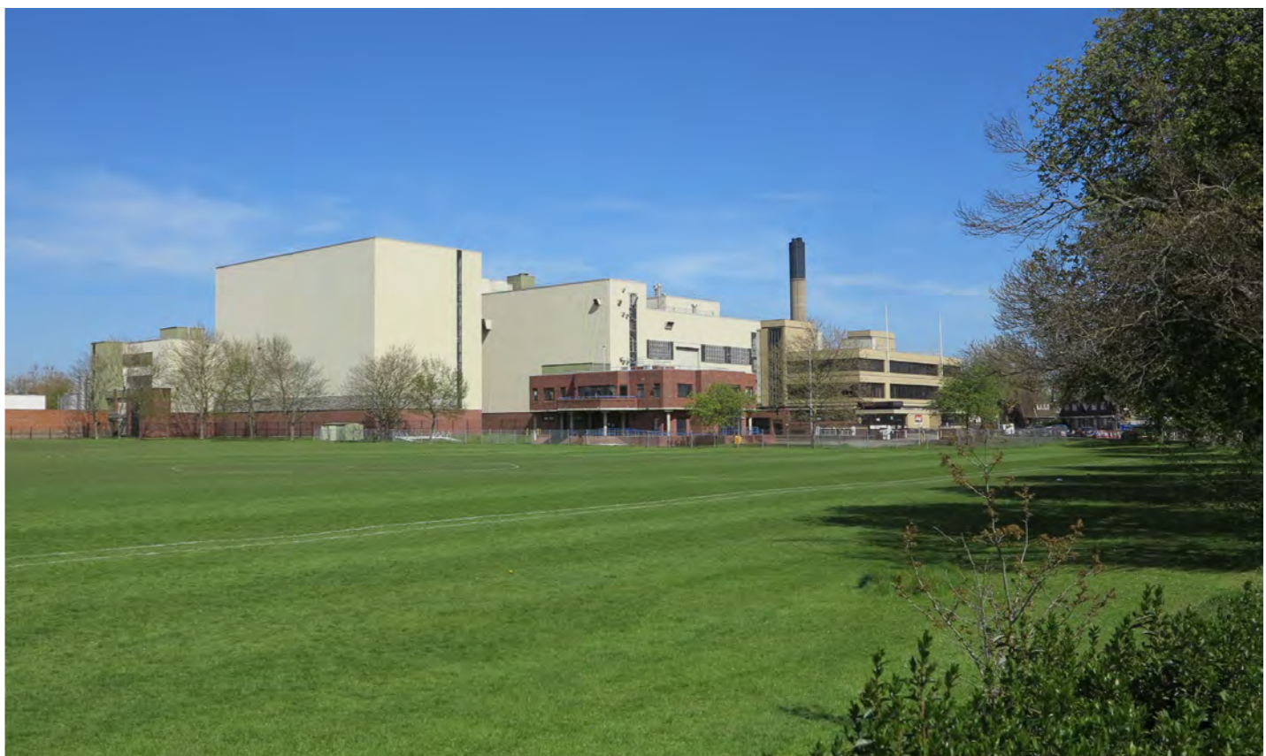
Existing Brew House industrial buildings
