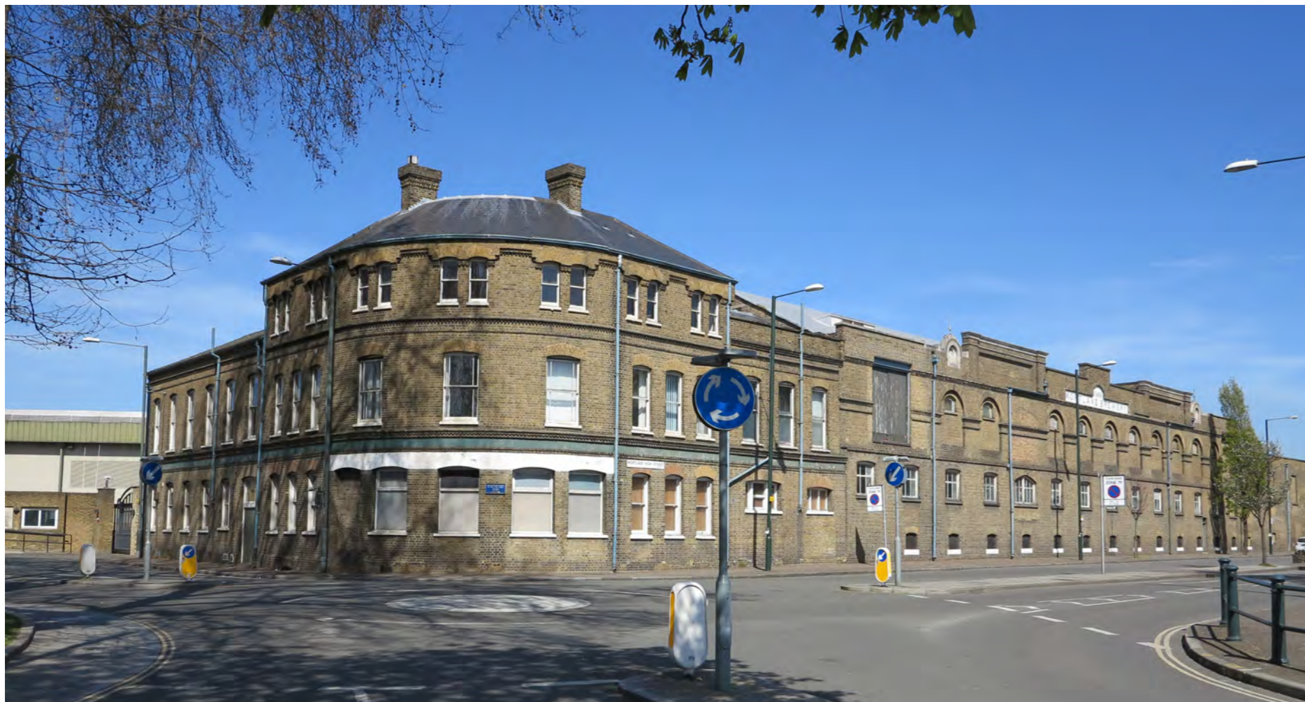
Existing former hotel and bottling building
