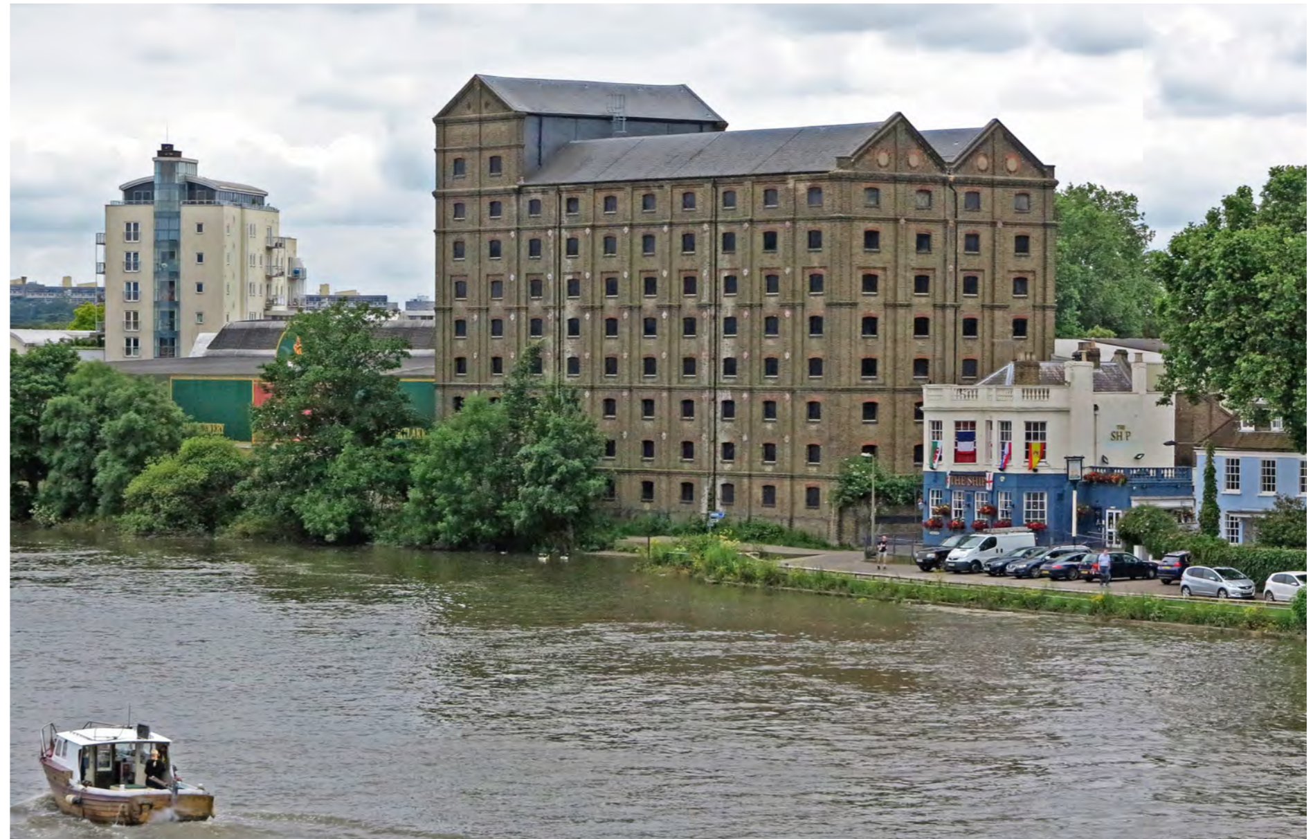
Existing former Maltings Building
