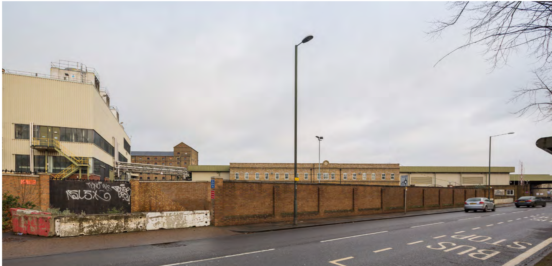
Existing view of site from Lower Richmond Road
