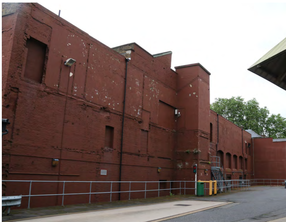
Existing north elevation of former bottling and hotel building.
