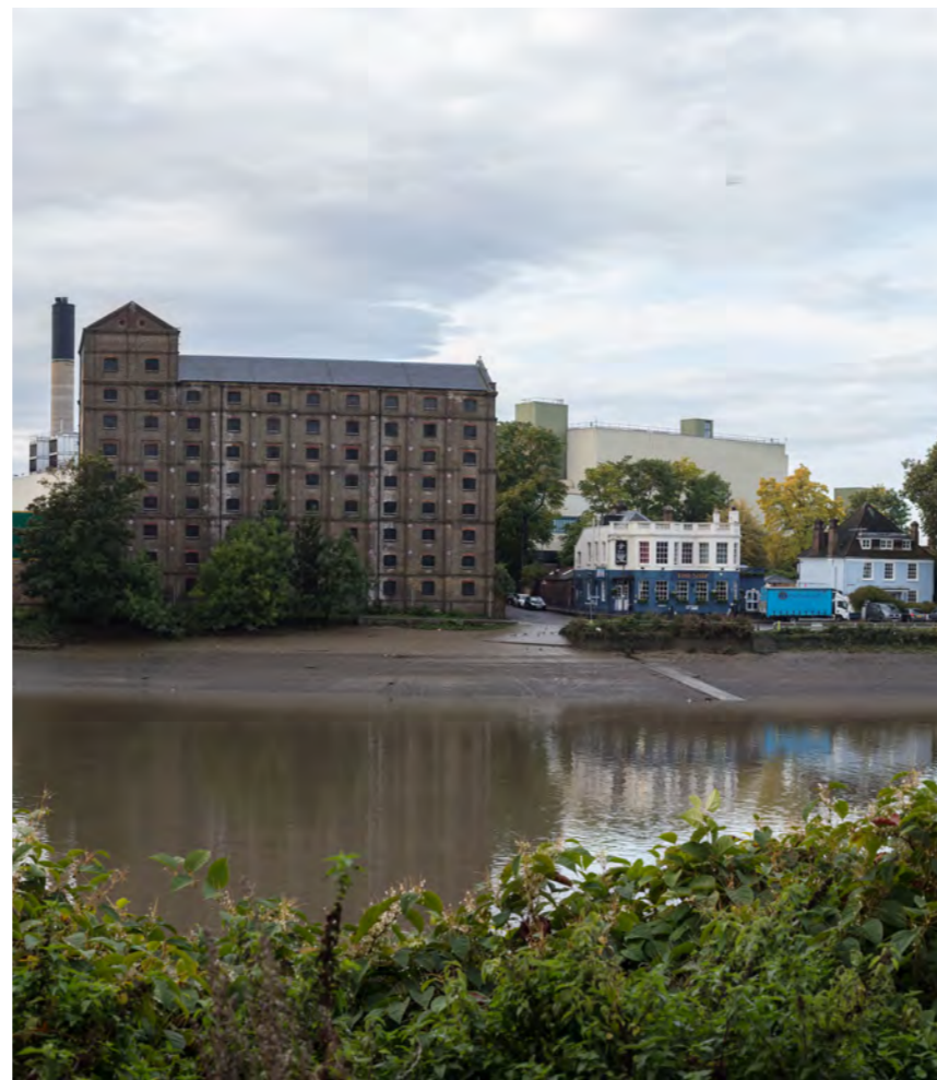
Thamesbank river frontage (with former Maltings building to the left)
