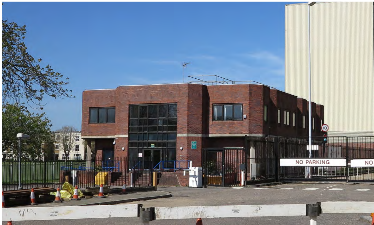
Existing Sports Club building
