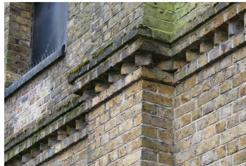
Dog tooth brick detail to Maltings facade
