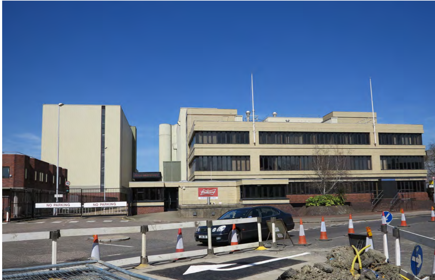
Existing office block
