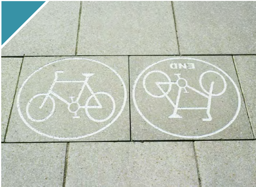
Artificial Stone Flag Paving
