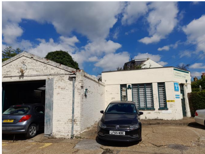
Photograph 3 Hardstanding and Building Group G4
