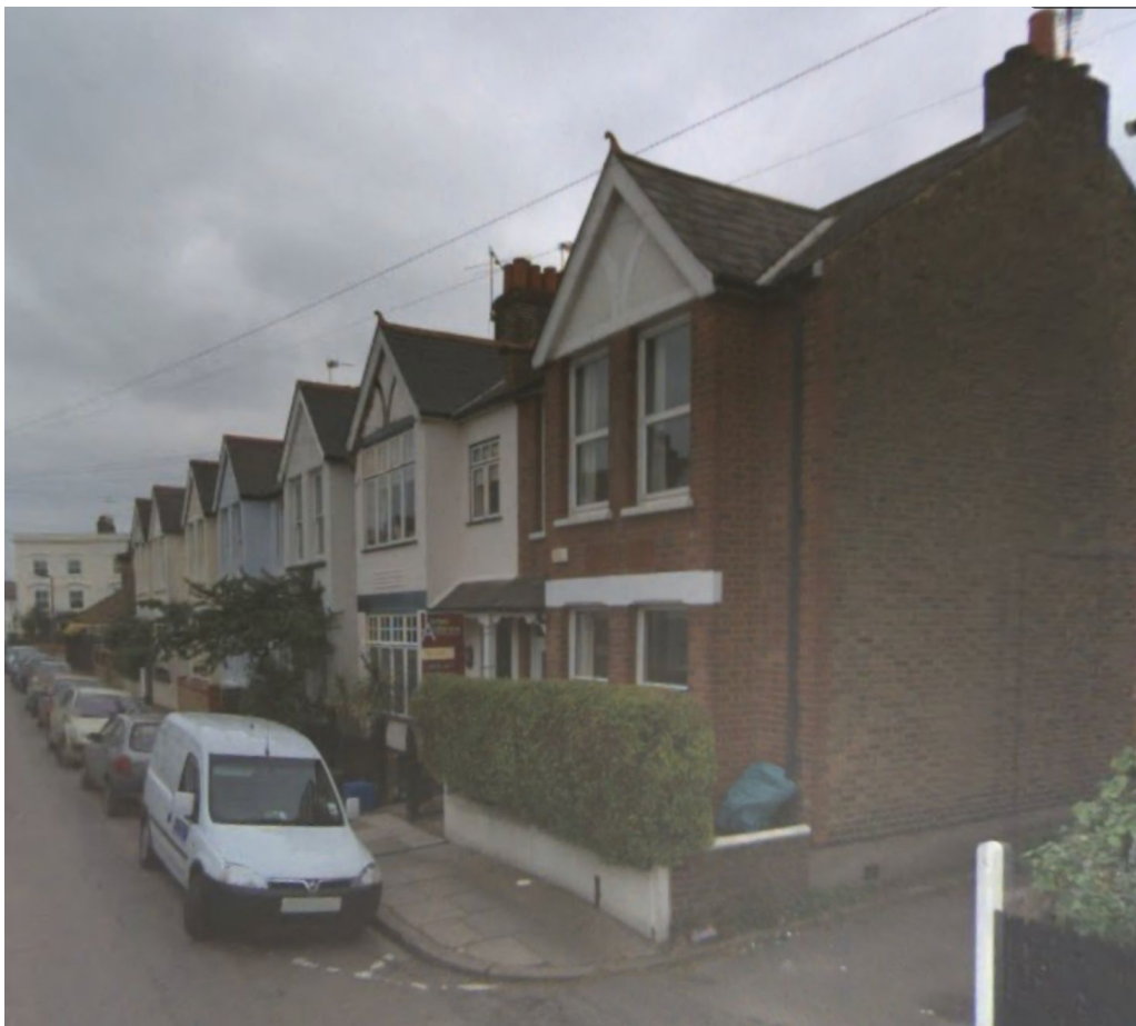
16, 18, 20 and 22 Fitzgerald Avenue
