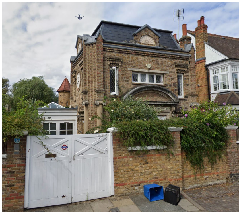
1a Fitzgerald Avenue
