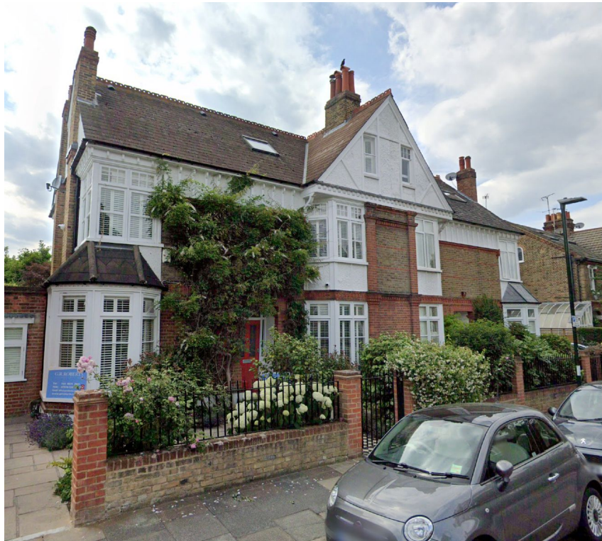
3 and 5 Fitzgerald Avenue
