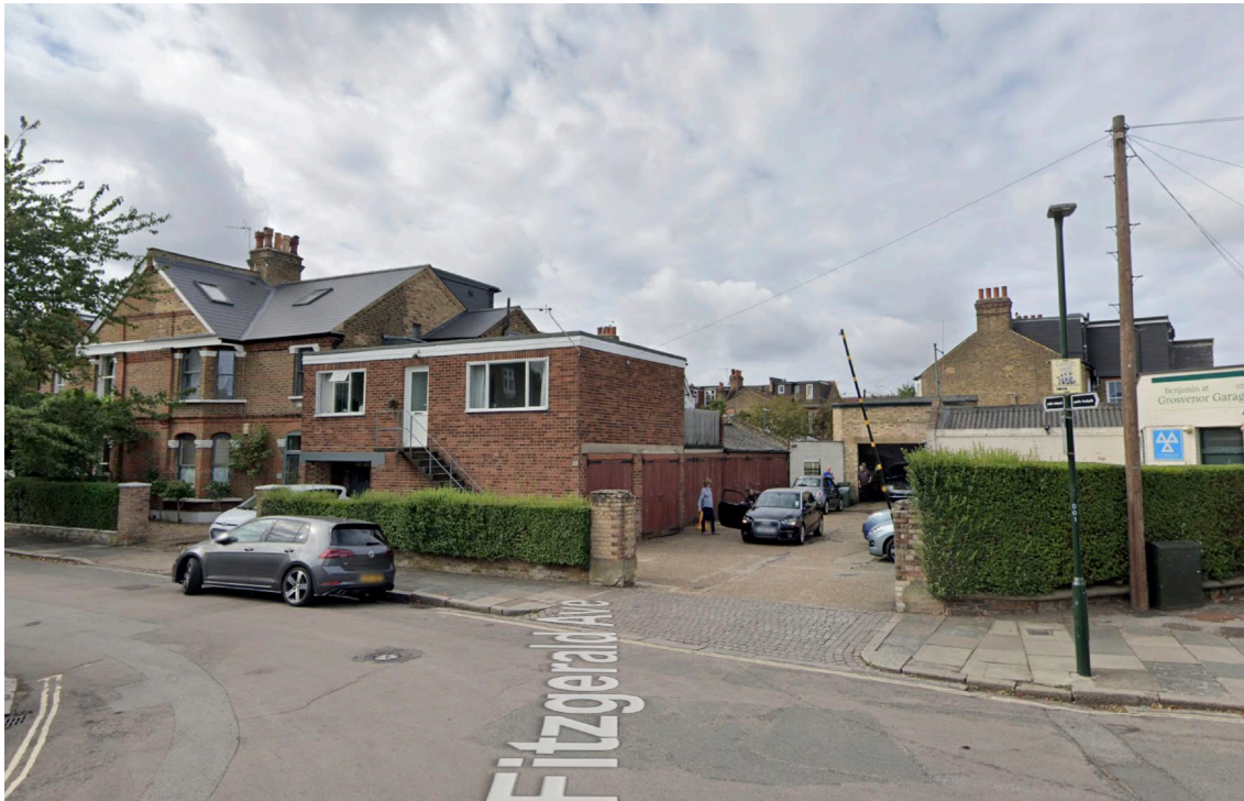
Existing Buildings on Site
