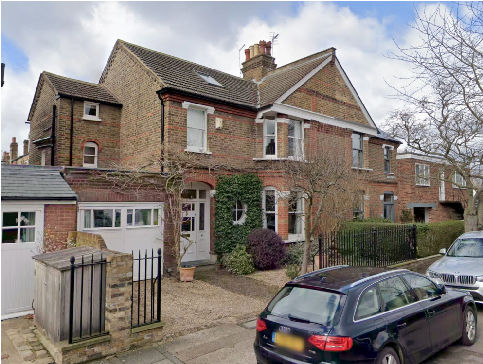
11 and 13 Fitzgerald Avenue
