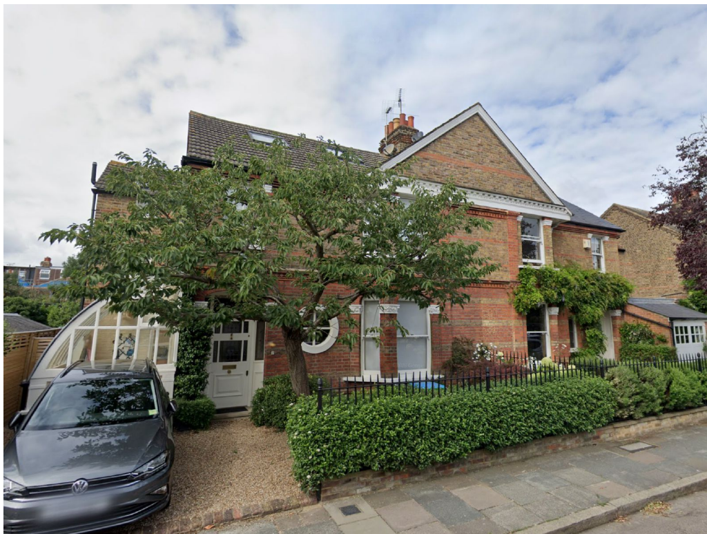
7 and 9 Fitzgerald Avenue
