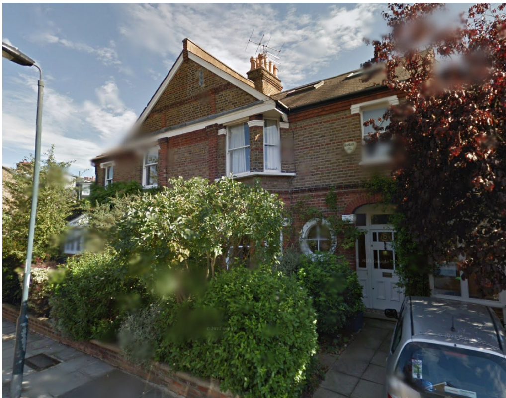
8 and 10 Fitzgerald Avenue
