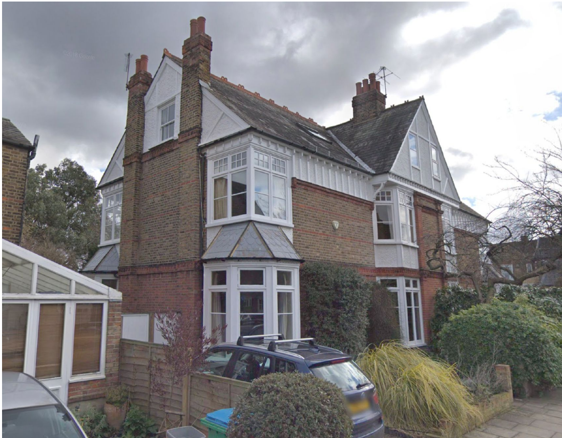
4, and 6 Fitzgerald Avenue
