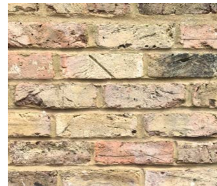
Yellow multi stock brickwork
