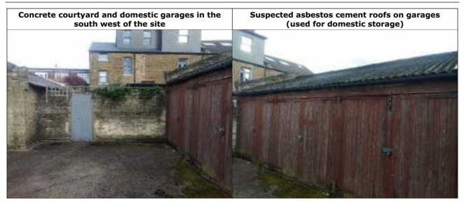
A further row of domestic garages is present along the southern boundary of the site. As with the other buildings on site, these were noted to have suspected asbestos cement roofs. A flat was present above the eastern garage. The garages were used car parking and domestic storage.
