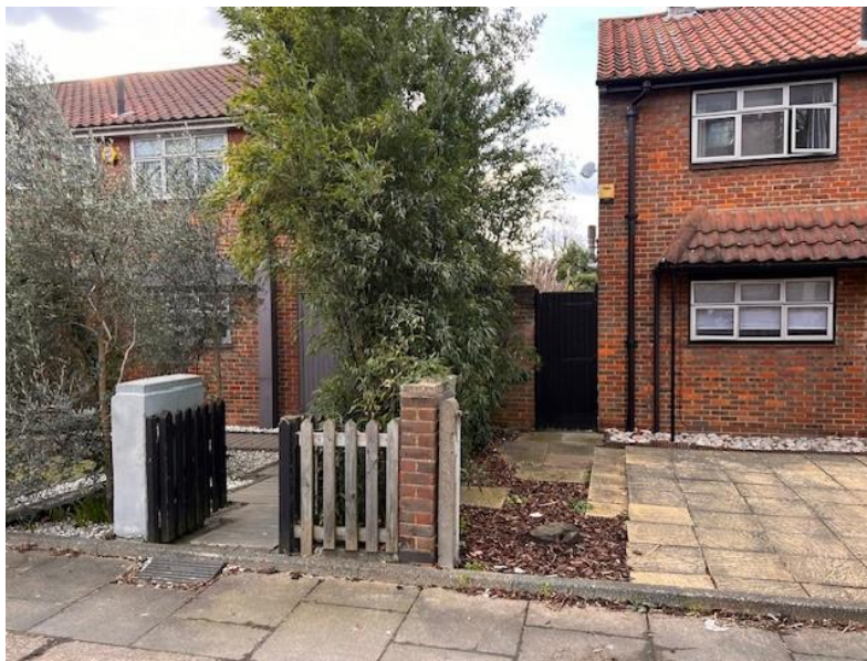
Above. View of front elevation and boundary with No.397
