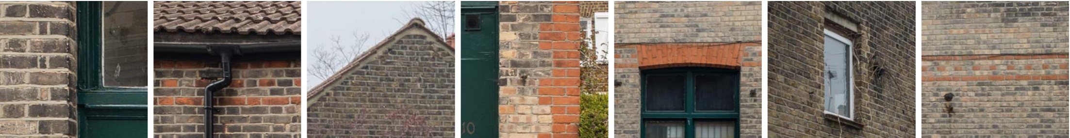
Darker buff coloured brick to window reveals. Green painted timber windows.
