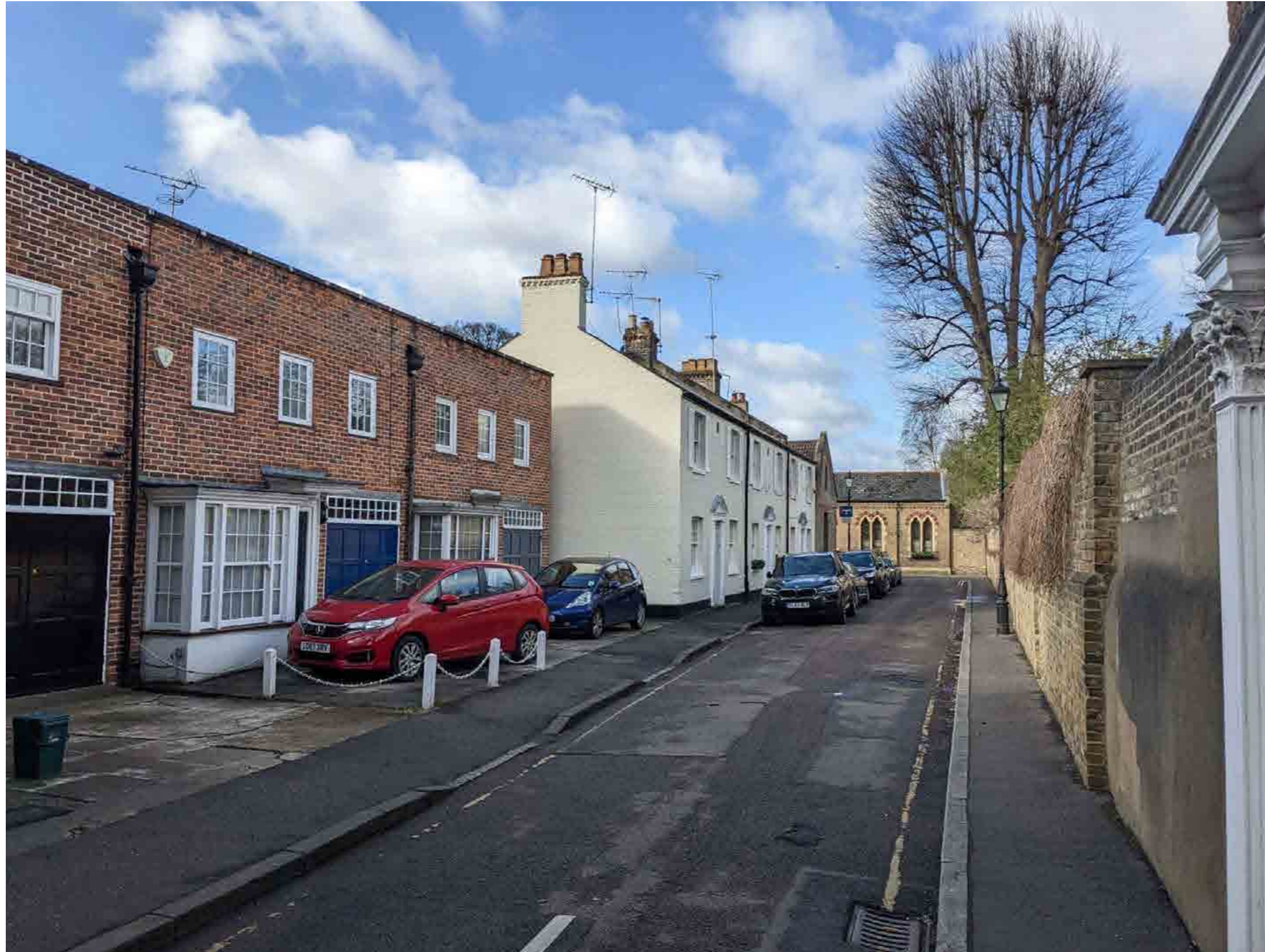
Streetview of the existing building looking west
