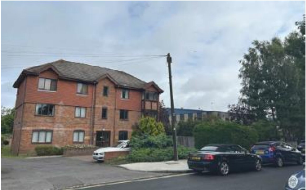
Figure 2: Adjacent Ryedale Court
