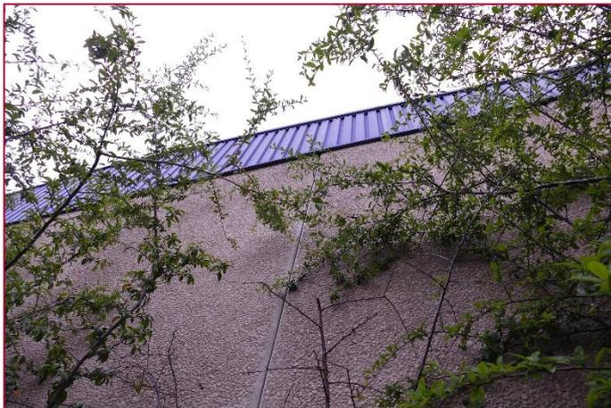
(c) Metal fascia feature at wallhead. Tightly sealed to the wall.
