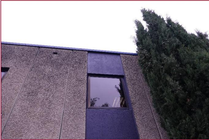
(d) Metal batten around top of wallhead. Apparent gap above window panels, but no PRF created here.
