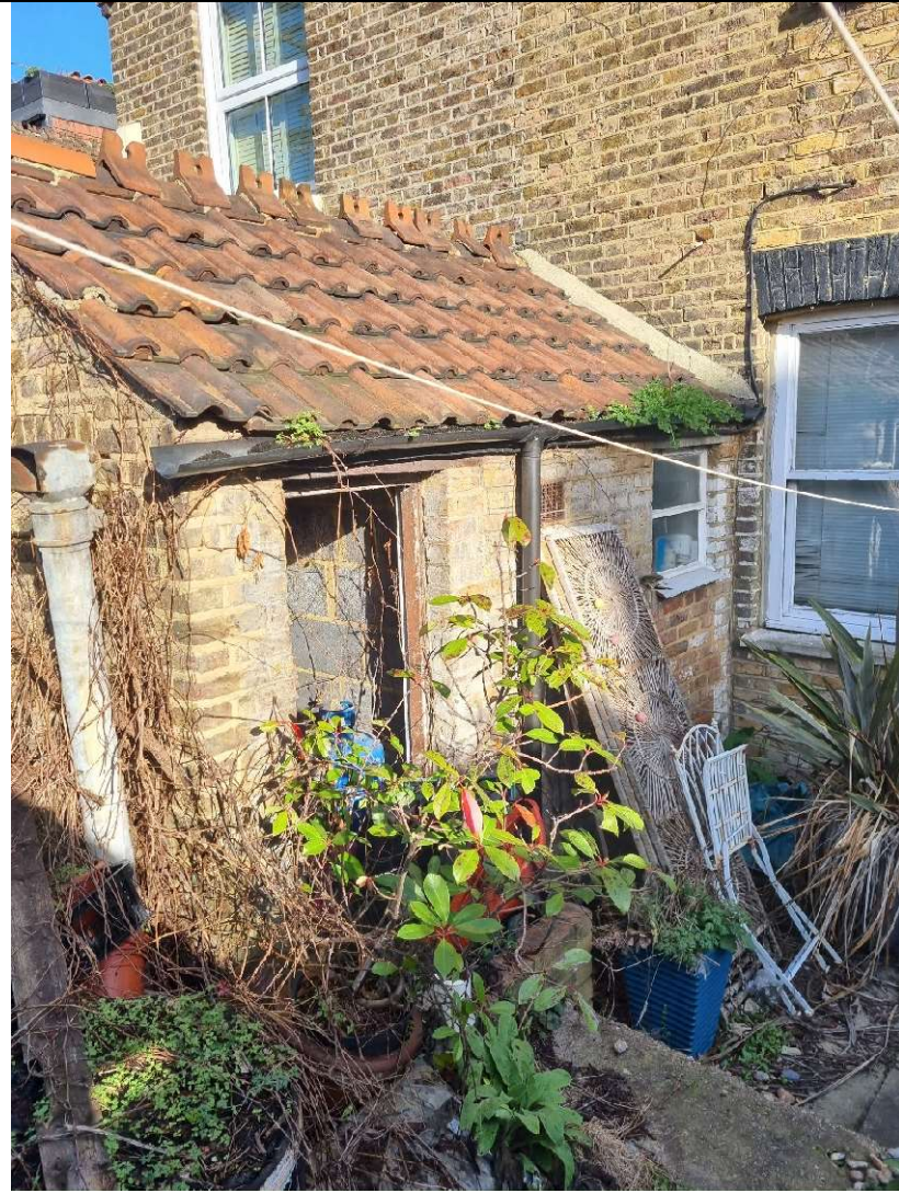
5.4 Existing out-building to be demolished.
