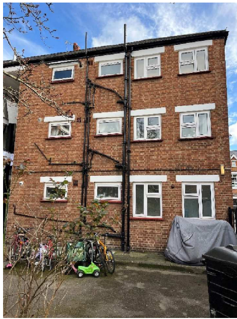
Photo 06: Side elevation taken from the rear of Ashleigh House, looking East
