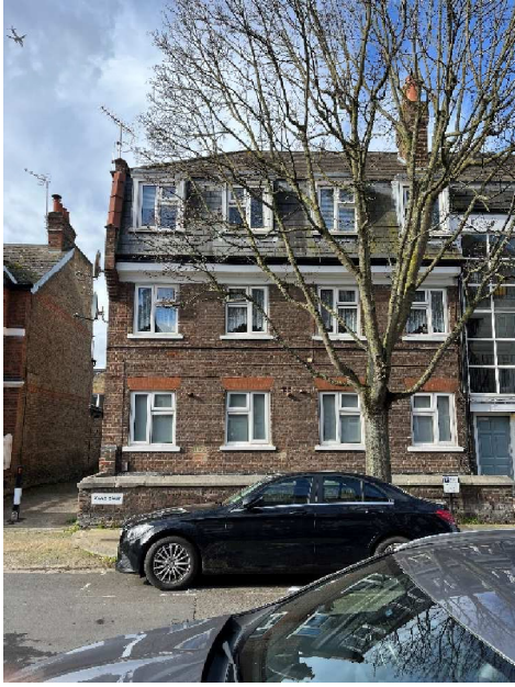
Photo 05: Side elevation taken from Ashleigh Road
