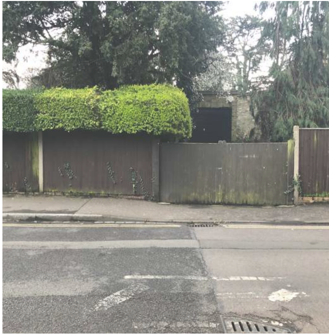
Image: Roadside view of gate
