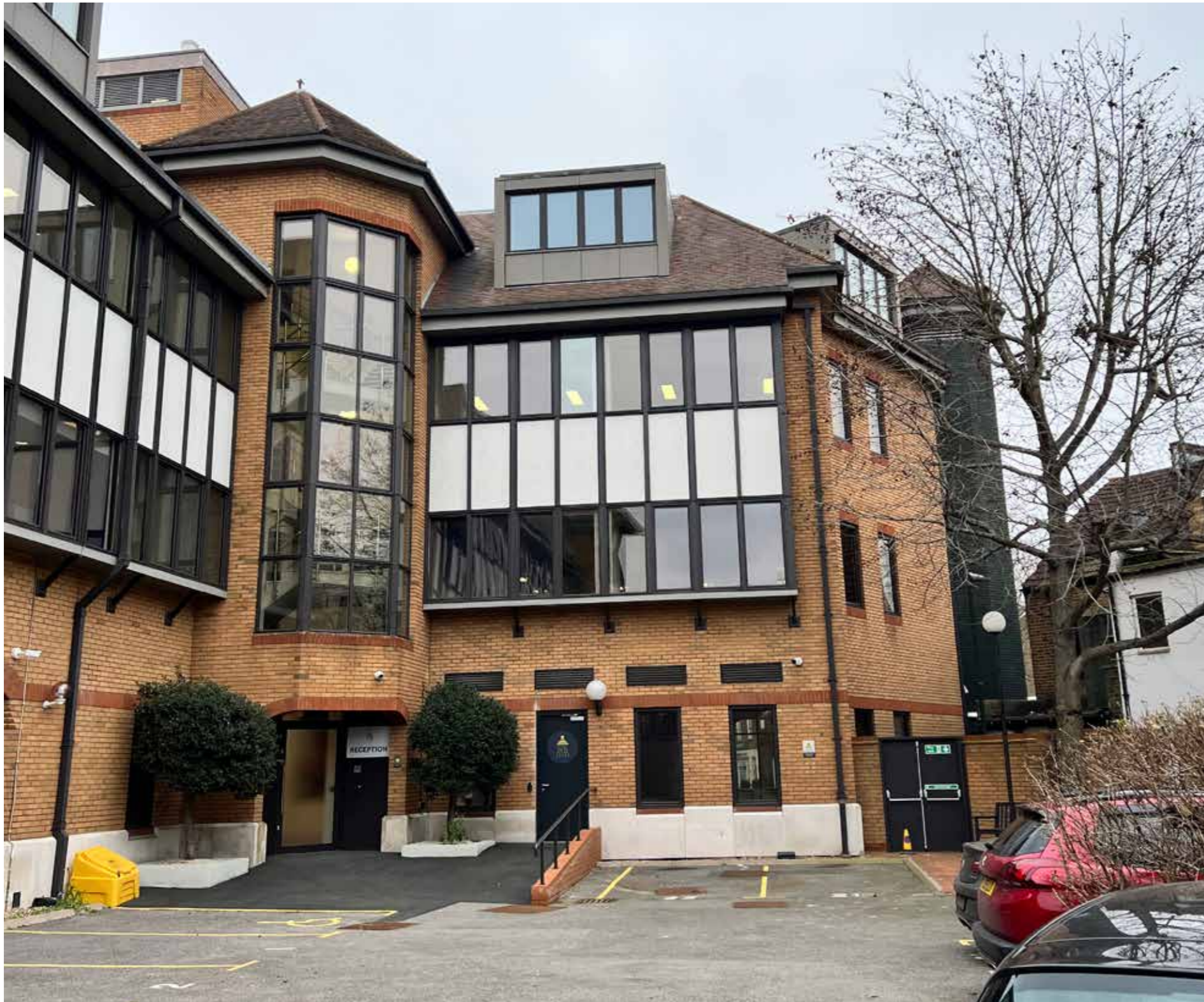
The current car park performs as an accessible route into the building
