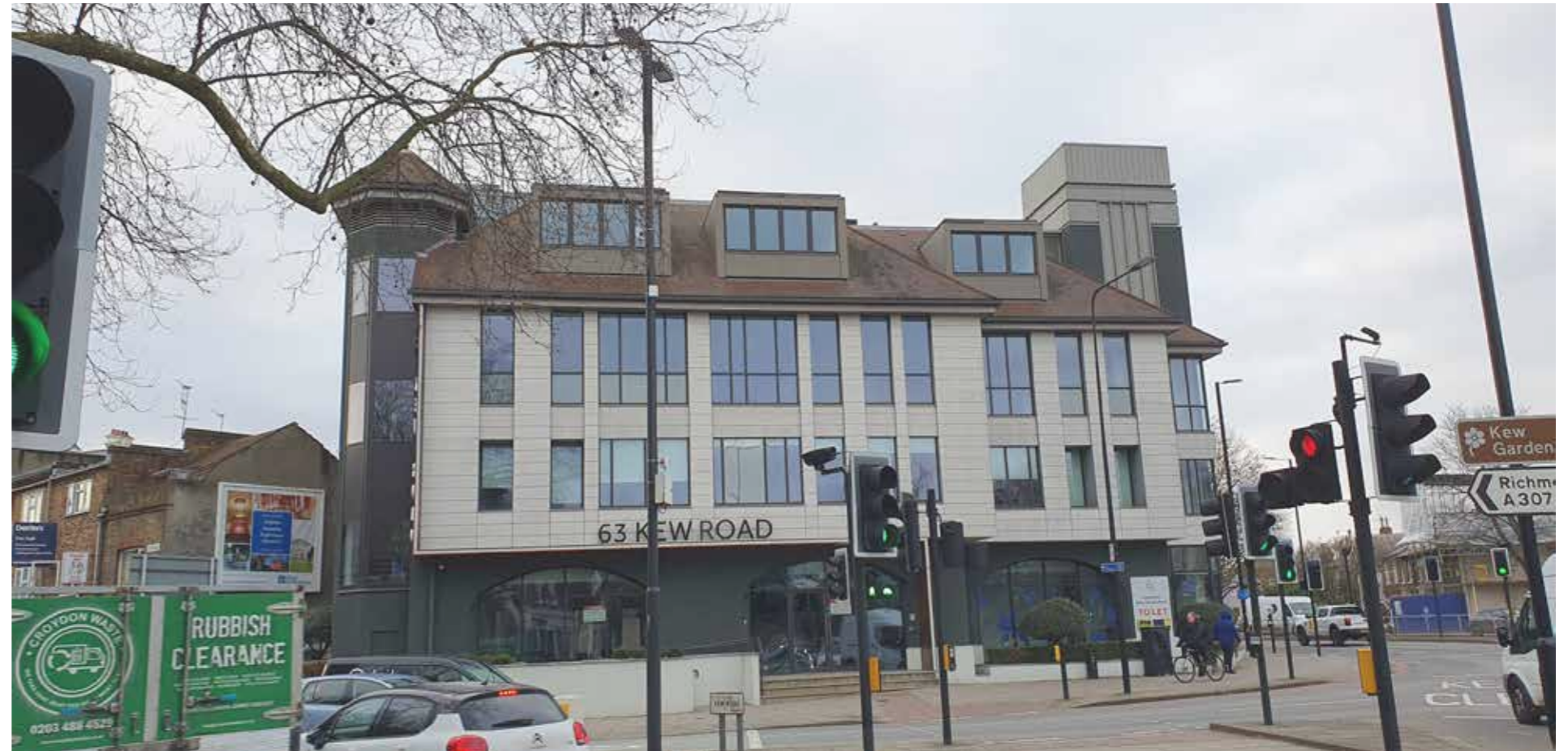
Existing office building
