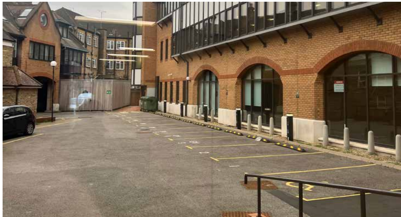
Existing car park areas
