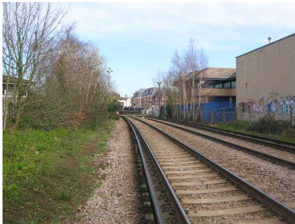
View from far-side cess, with site to the right
