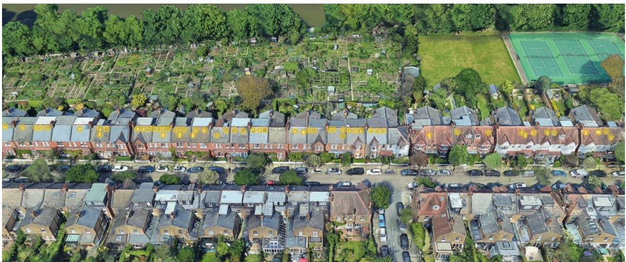
Aerial Photograph highlighting the prevalence of roof lights on the front façade.
