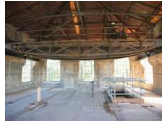
Top level 3 of the western block, 'The Beam,' with a large steel gantry crane and steel trusses
