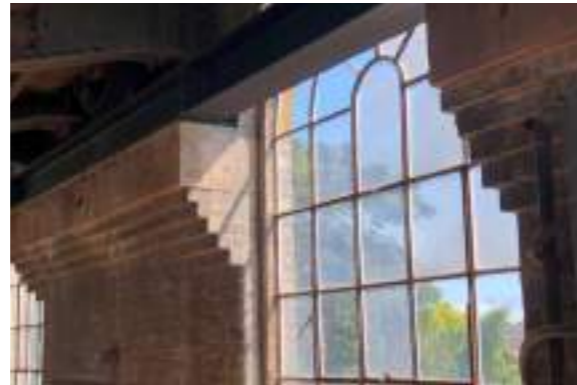
Interior of the western pump house of Karslake building
