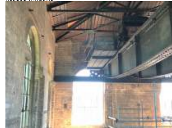
Top level 3 of the western block, 'The Beam,' with a large steel gantry crane at the right
