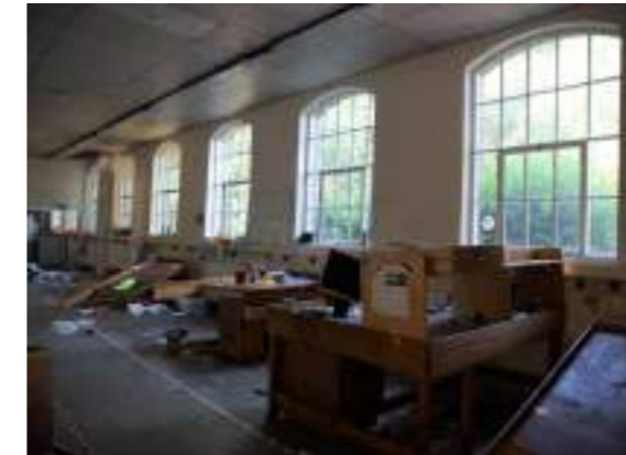
Interior of the single storey block, previously used as office space
