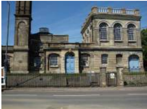
Pedestrian entry off of Lower Sunbury Rd
