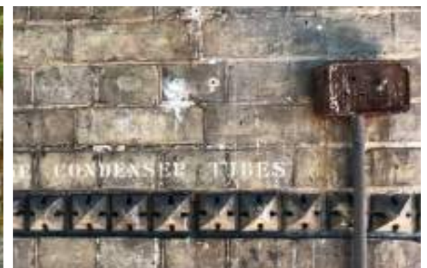
Dog-tooth detailing set within the walls
