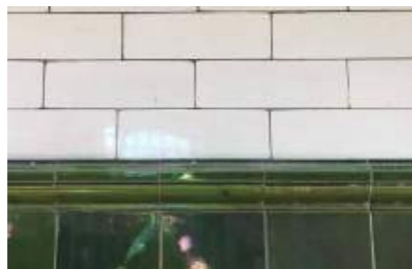
White and green Victorian glazed ceramic tiles can be found in good condition - to be retained and cleaned
