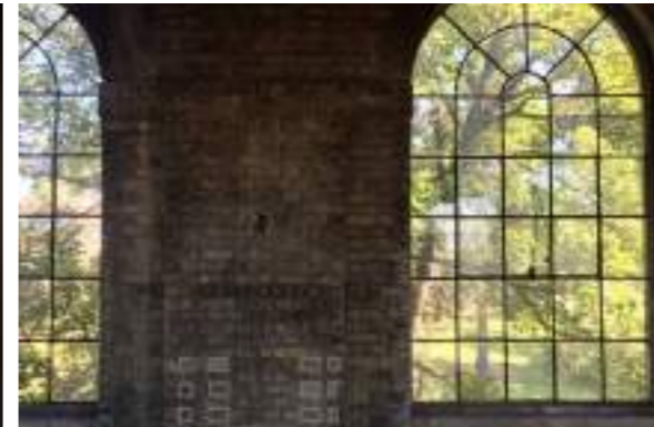
The Beam's second storey with cast-iron round-headed windows
