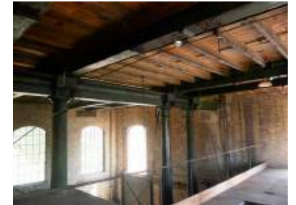
Tuscan order steel columns hold up the second floor's large steel beams in The Beam
