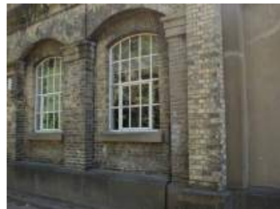
A majority of the existing windows are not original, they are more modern replacements
