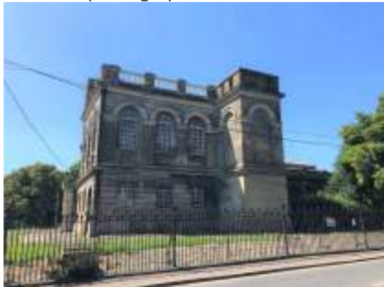
Large pump house on the northeast corner
