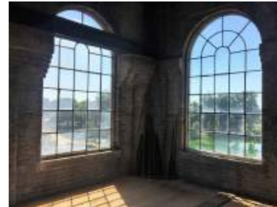
Top level 3 of the western block with original, round-headed windows
