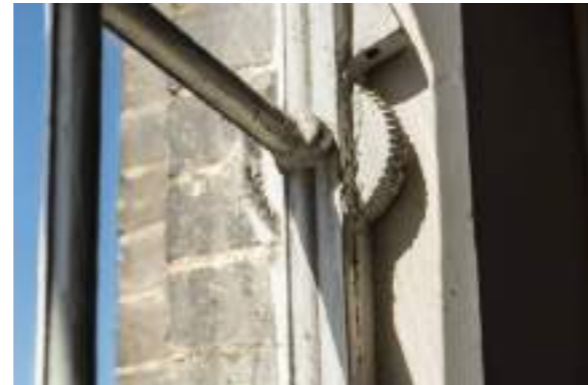
Original window opening mechanism
