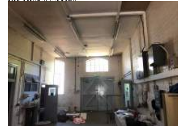
The central block has been subdivided with concrete block and aluminium partitions in the late-twentieth century
