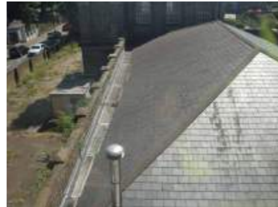
View from the western block, looking over the slate roof of the central single storey block
