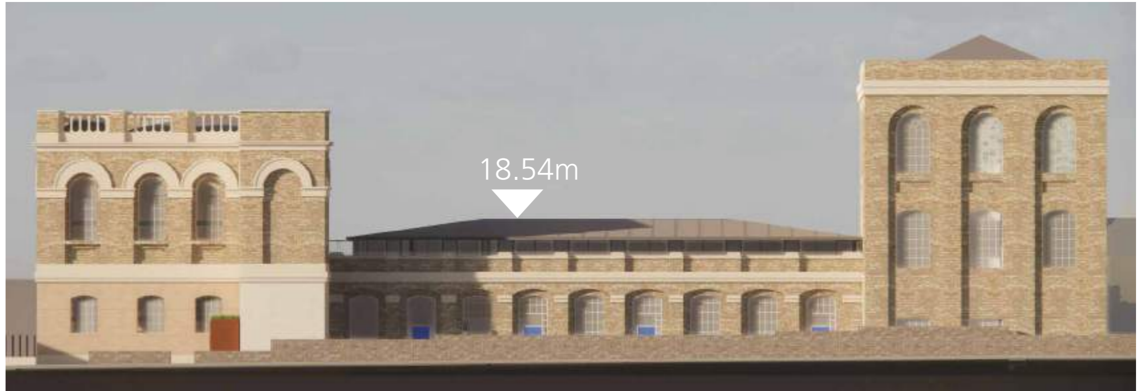
Updated roof extension
