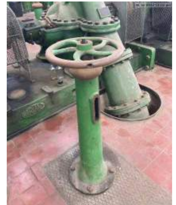
Valve Control standard for centrifugal pump Date: 1932 Size: 0.4 d Report comment: Low to medium significance
