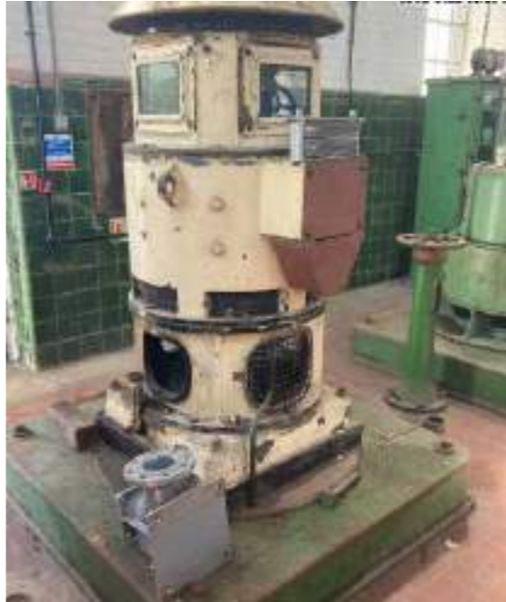
Replacment W H Allen DC motor Date: Undated Size: 1.6m x 1.6m Report comment: Low to medium significance
