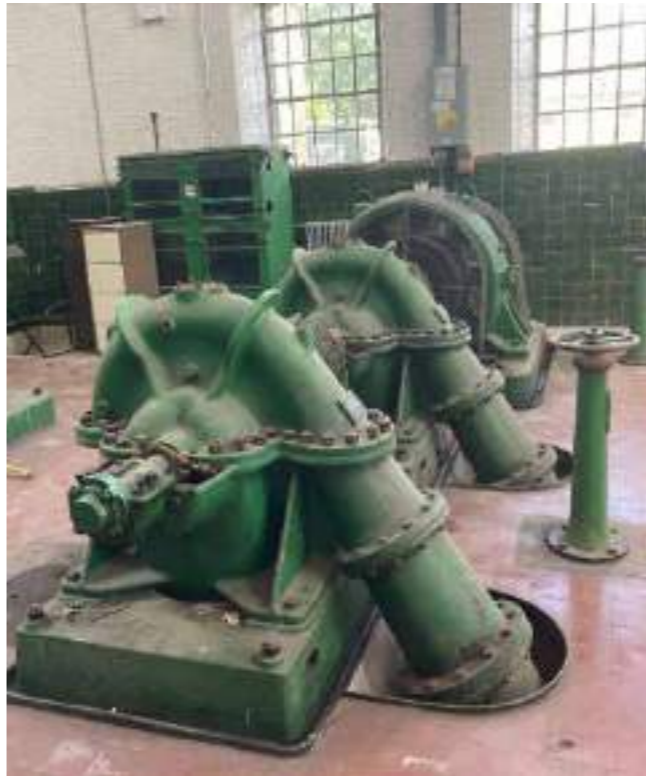
Harland twin impellar electric centrifugal pump set Date: 1932 Size: 5.8m x 2.5m Report comment: Low to medium significance
