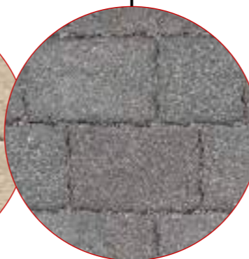
Shared Roadway Permeable block paving colour or size to be used to denote vehicle movement lines while providing pedestrian priority across the site.
