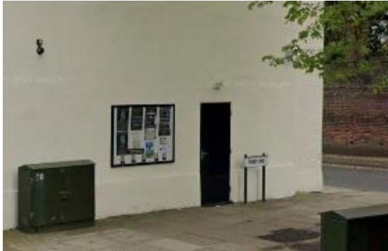
Figure 3 - fire exit door on Sandy Lane (N) elevation
