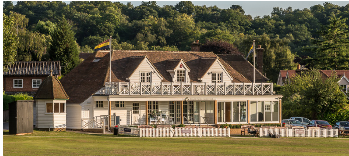
Reigate Priory Cricket Pavilion
