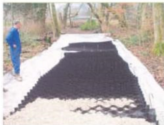
CellWeb during installation.
