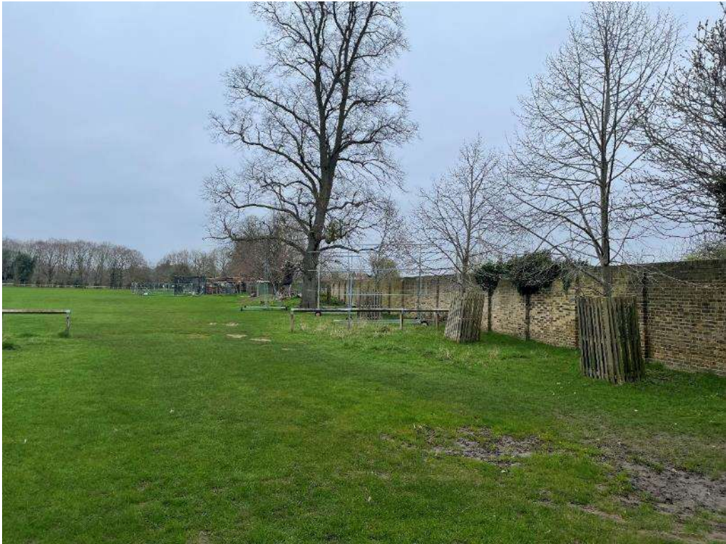
Figure 3.10: Photograph of the Site and burnt-out pavilion building as seen from the south (Church Grove path) and with the high brick boundary wall to the neighbouring allotments visible to the right
