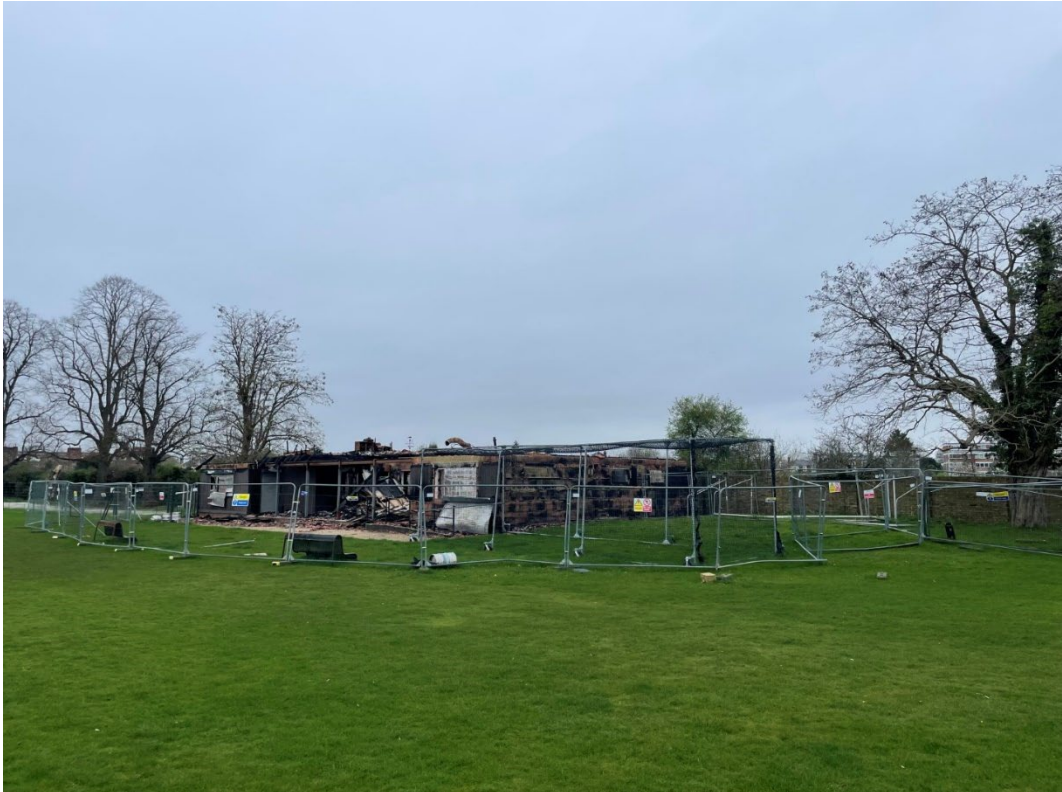
Figure 2.3: Remnants of former Cricket Pavilion damaged by arson attack
