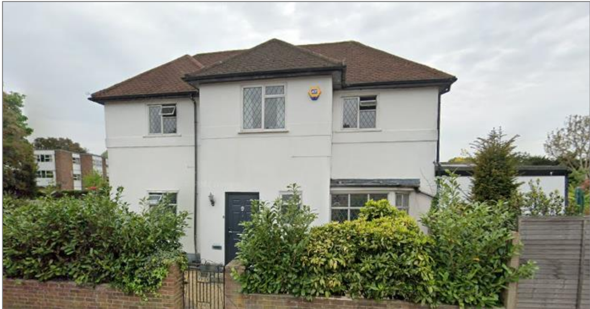
Photograph 1: The site as viewed from Links View Road.
