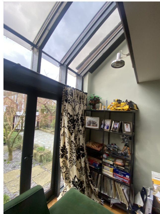
Photograph showing existing single-glazed 'conservatory' structure
