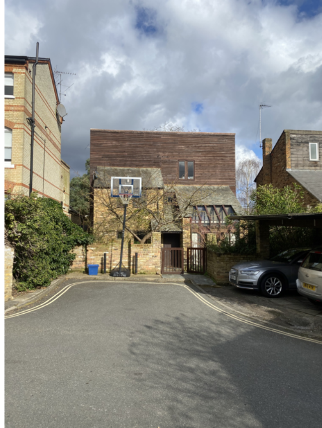
View from Rosemont Road showing relationship with neighboring properties
