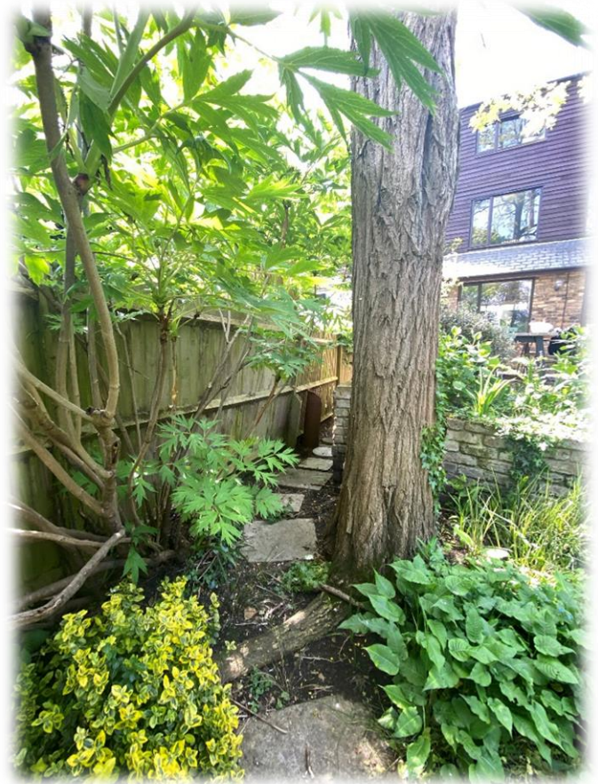
False Acacia (T1) Mature Surface Root with Upper Surface Damage and Decay
