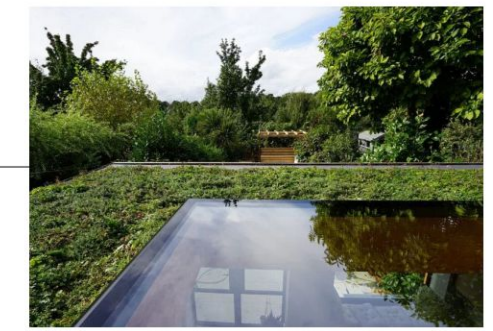
Green sedum roof covering
