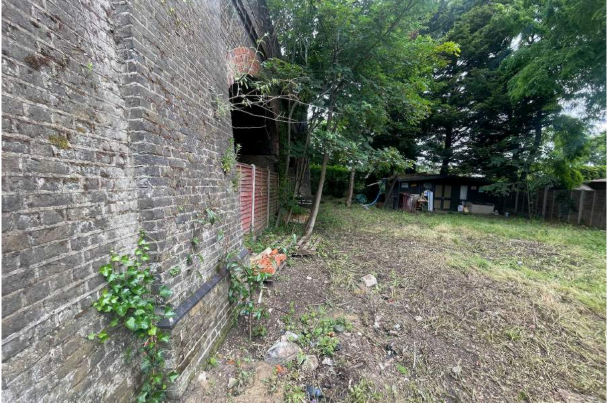
7 - Western Boundary Facing North
