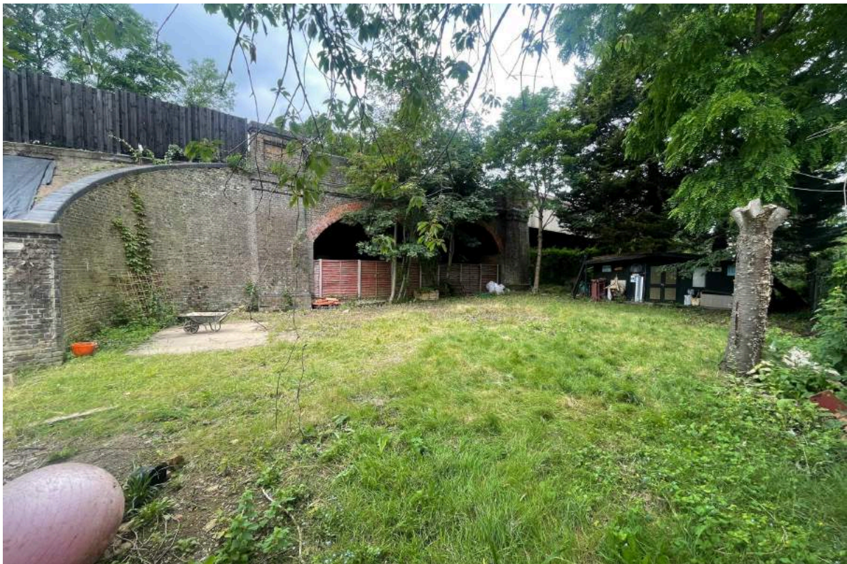
2 - South-Eastern Boundary Facing North-West
