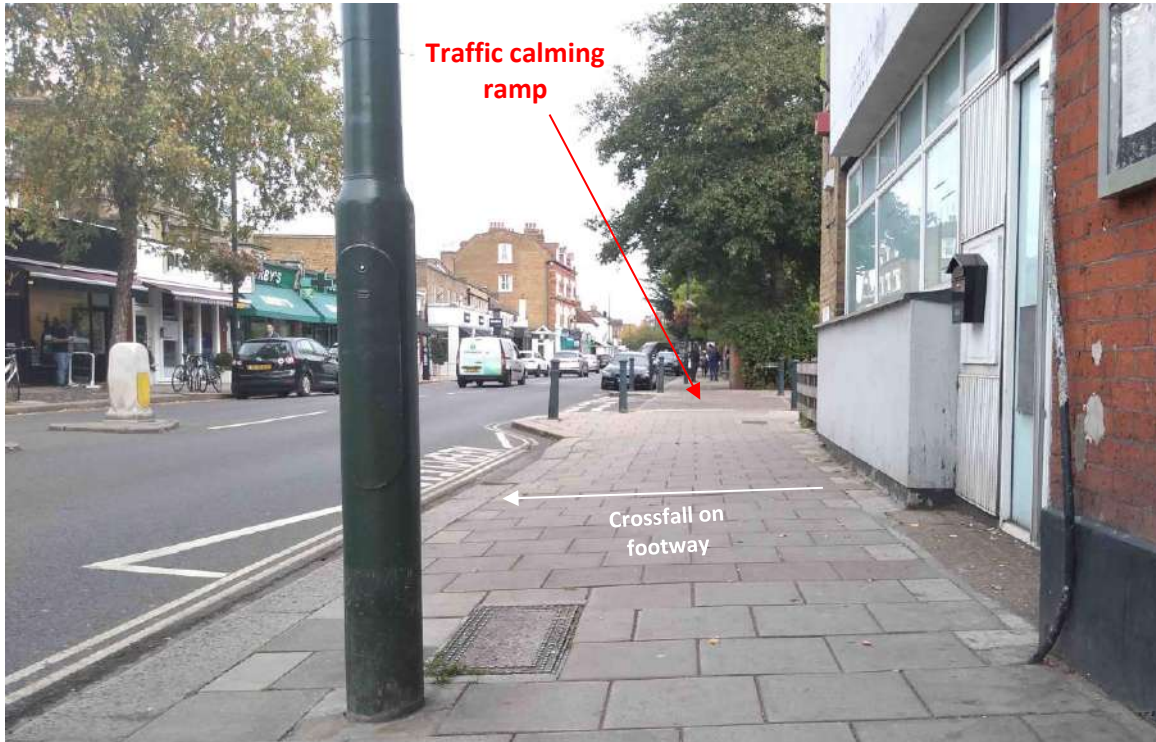
Photo 3: Gentle crossfall on High Street footway to front of No.42.
