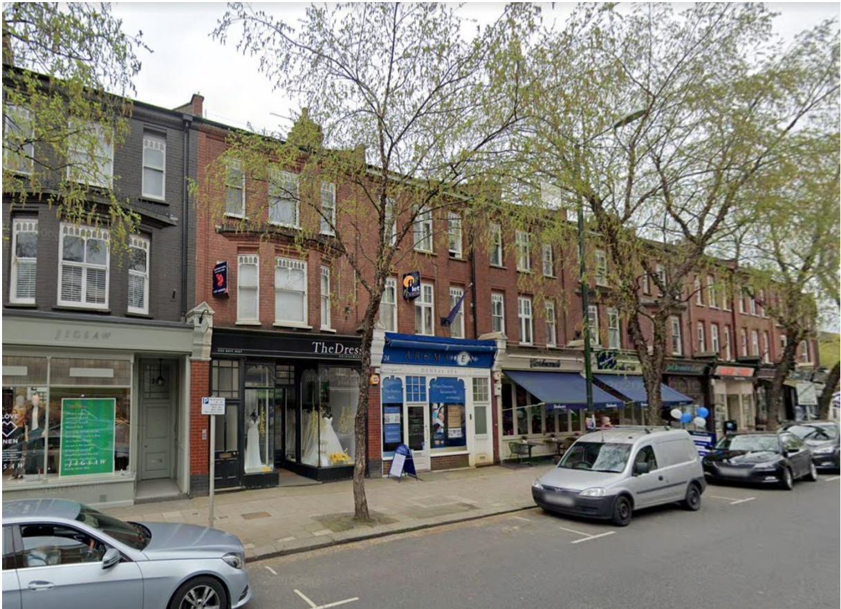
Figure 2.13 Part of the parade of Nos 10-36 High Street, built in c.1903 (Google Streetview, 2018).
