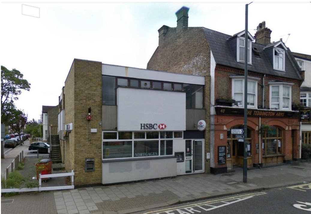
Fig. 2.10 The existing building at No 42 High Street during use as a bank (Google Streetview)
