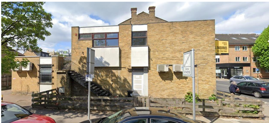
Figure 5.2: The Cedar Road elevation of the Site as existing
