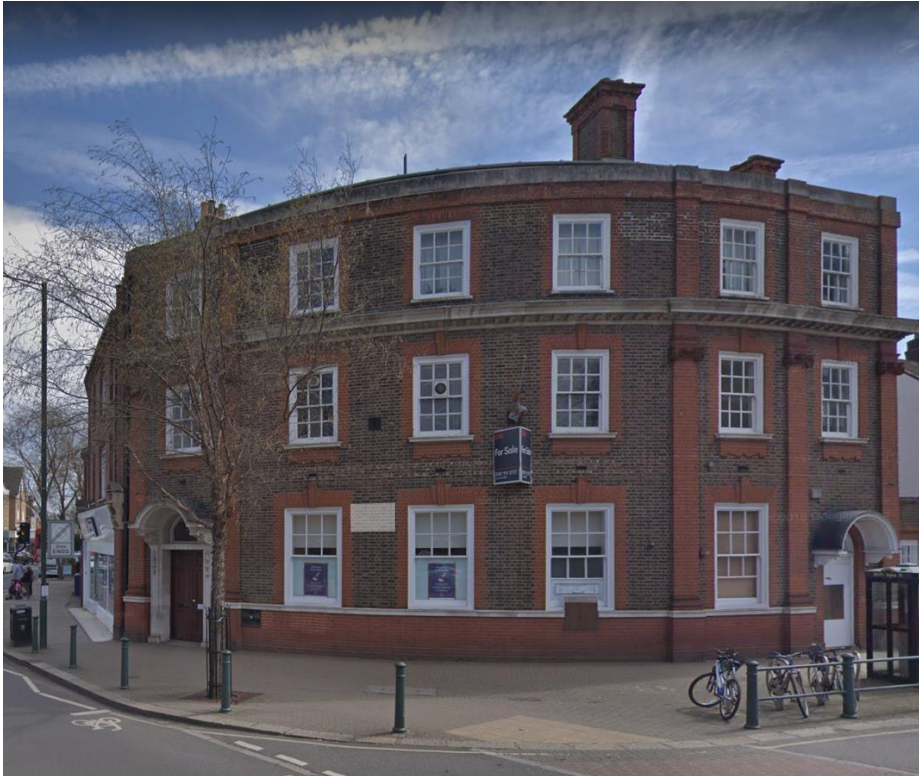
Figure 2.14– Former NatWest Bank, 6 High Street, built in c.1909 (Google Streetview, 2018).
