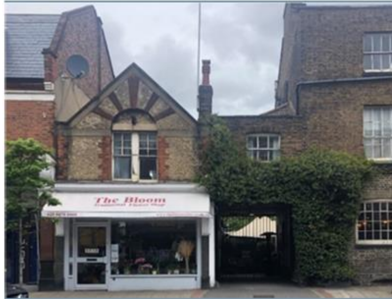
Carriage Entrance & Adjoining Commercial Unit
