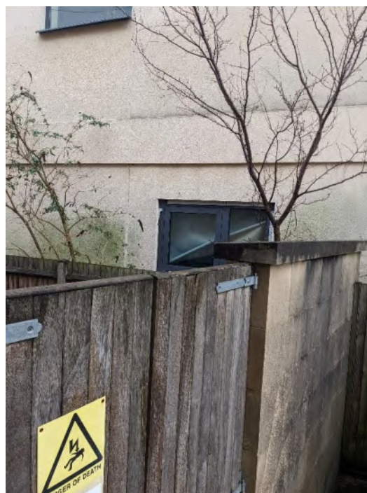
Figure 04 – Ground floor west-facing window
