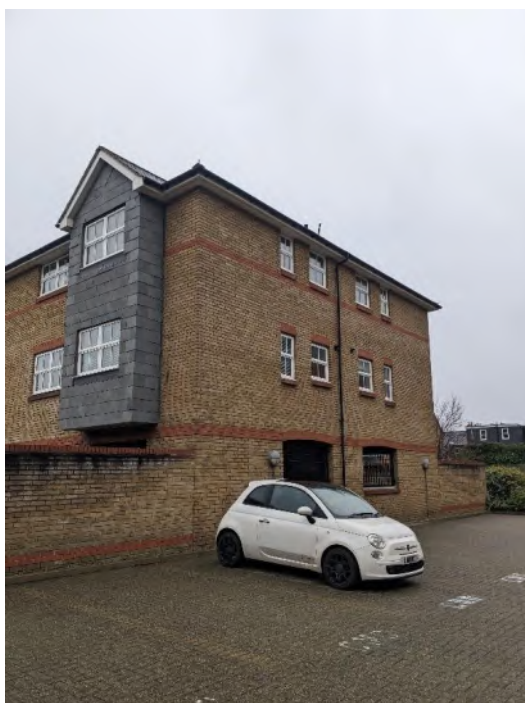
Figure 05 – 1-16 Tersha Street north flank
