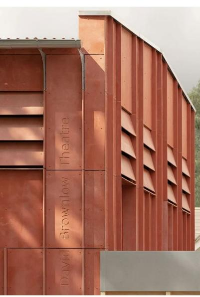
It is important for the scheme to source sustainable and environmentally friendly materials that also sit well against the existing building. Viroc is a fibre cement board that is a natural facade solution with a wide variety of applications. Combining the strength and durability of cement with the flexibility and workability of wood. The Viroc board is a composite material, created from a compressed and dry mixture of pine wood particles and cement.
