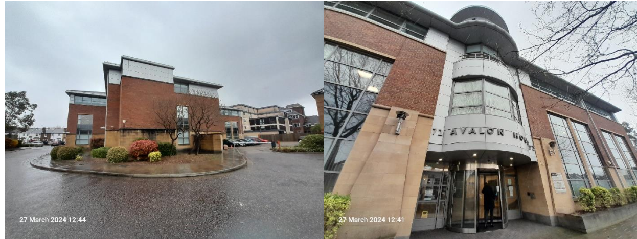
The majority of the site is hardstanding with sparse vegetation (left) and the one commercial building (right).
