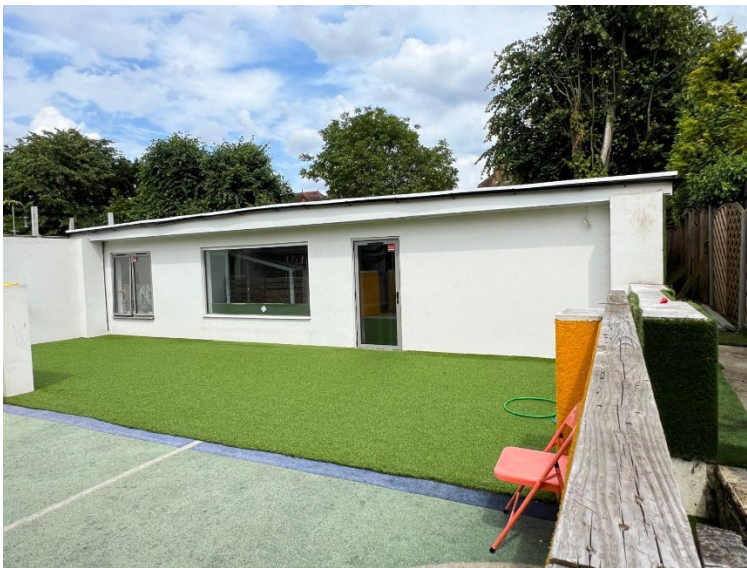
Existing outbuilding within rear of no.54 Percy Road
