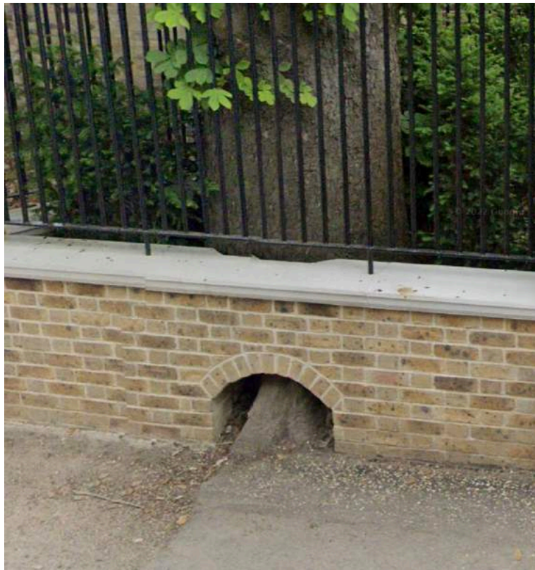
Tree lintel at 32 Fife Road
