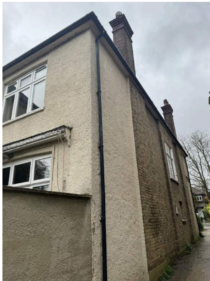
Existing render to rear and part of side elevation
