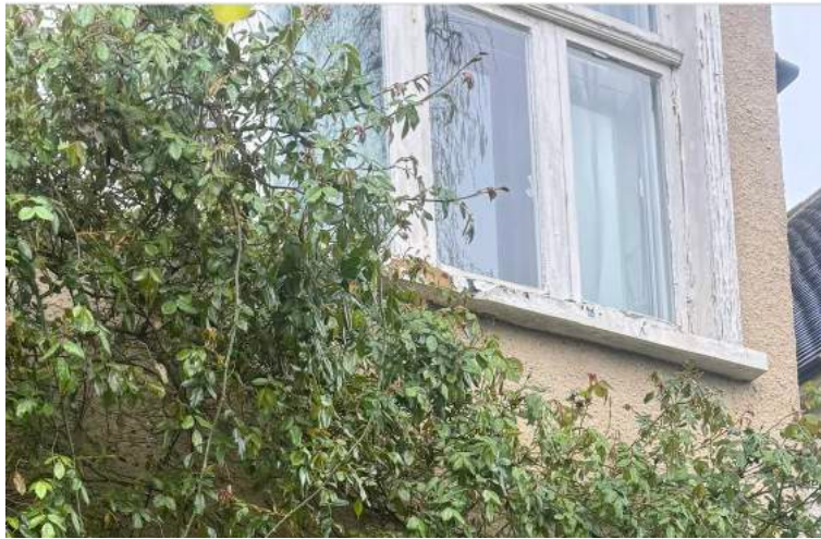
Existing protruding casement window frames
