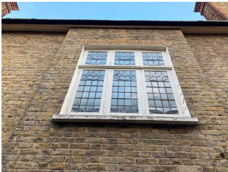
Staircase window to side elevation
