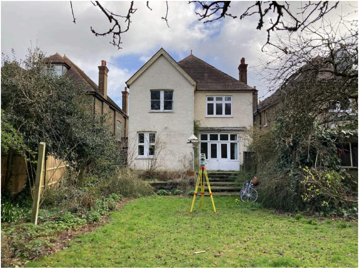
Existing rear elevation and stepped patio
