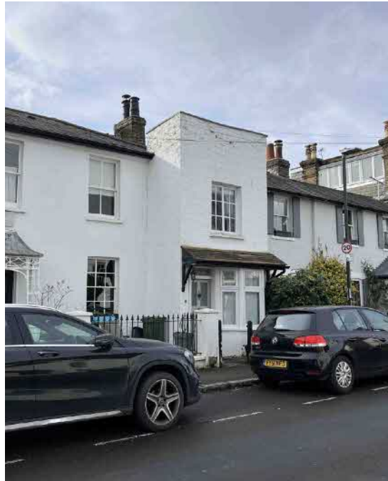
Street view showing No.51 Park Road
