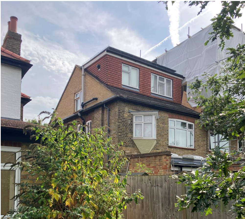
Rear Of 36 Taylor Avenue
