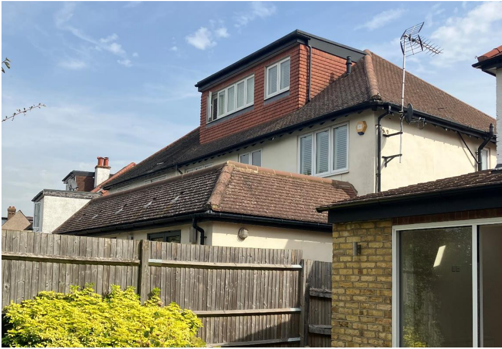
Rear Of 32 Taylor Avenue
