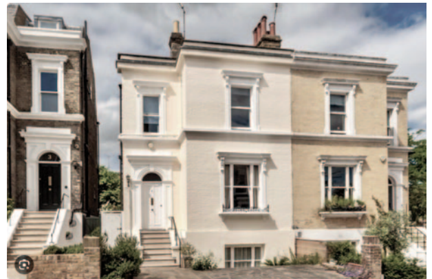
No 2 (painted brickwork) and on the right No 1 (cleaned gault bricks with coloured pointing). The form of their roofs is not visible from street level.
