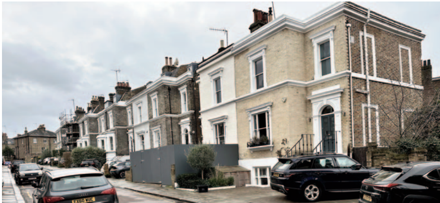
1 – 12 The Hermitage stepping up the hill. Nos. 1 and 2 in the foreground
