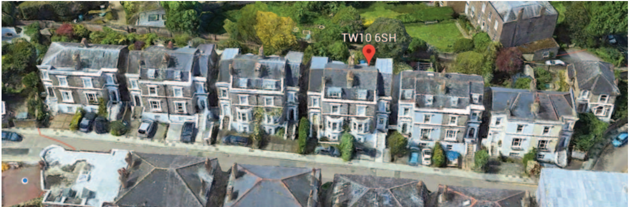
The group of paired houses, 1 – 12 The Hermitage stepping up the hill. The central group of four pairs is more coherent since the end pairs lack the matching Mansard roofs and have differing roof forms.
