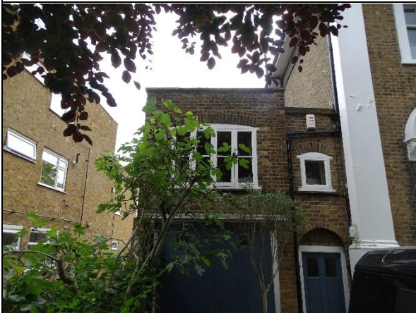
Photo 3: Main property with adjacent former coach house extension
