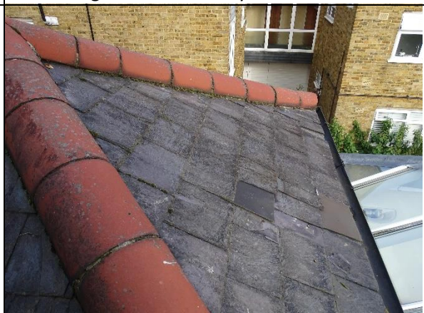
Photo 12: Southern face of former coach house roof with conservatory roof adjacent
