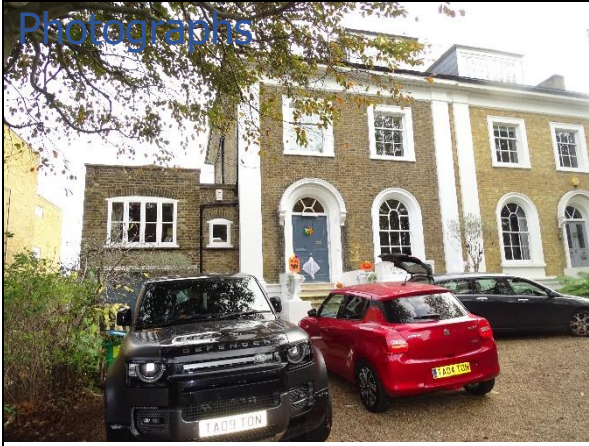
Photo 1: Front elevation of property showing gravel driveway and introduced shrub bed
