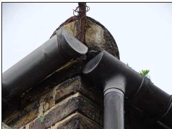
Photo 13: SW corner of roof showing concrete plug
