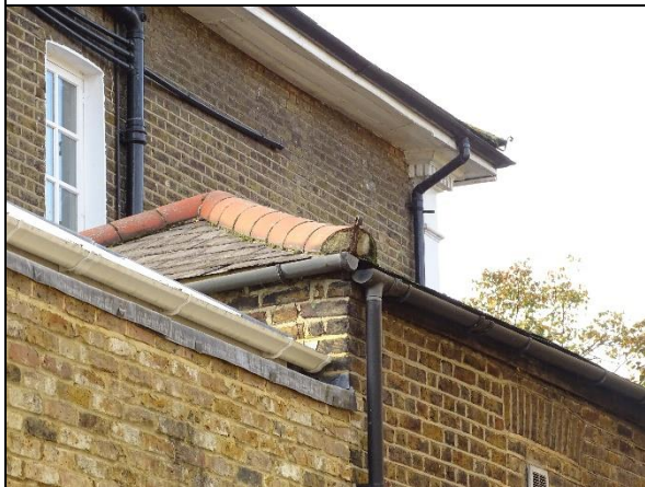
Photo 9: Northern elevation of former coach house
