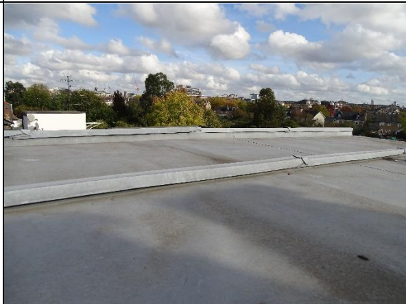
Photo 4: Flat roof of main building
