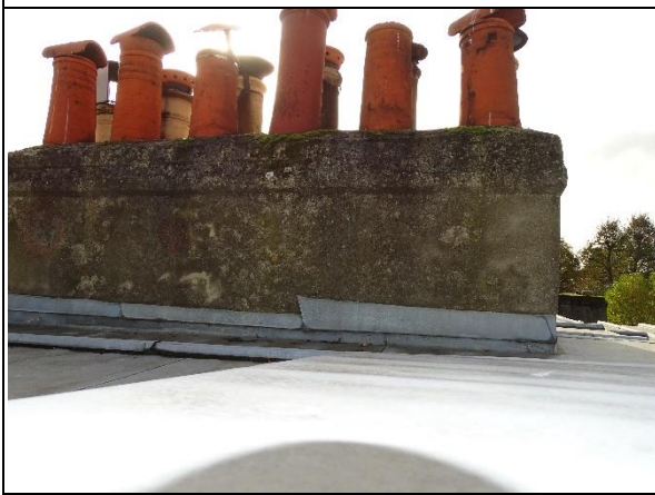
Photo 5: Chimnies on roof of main house
