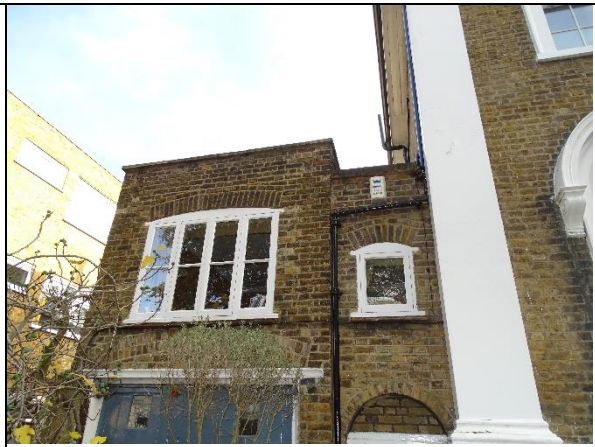
Photo 8: Front façade of former coach house
