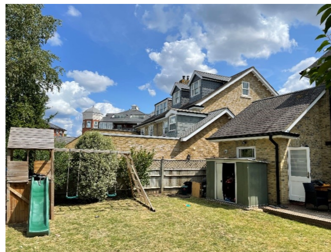
Fig 8 The rear elevation and neighbour (No. 11)
