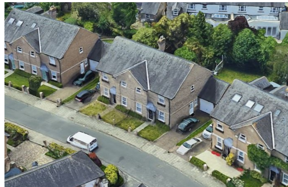
Fig 3 / This aerial photo illustrates the setting of the building toward the south-west end of the home. Additional glazing and room arrangement can help to create light, open spaces relating to the garden.
