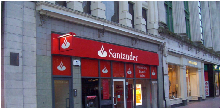
Basement damp proofing at Santander Bank, Marylebone
