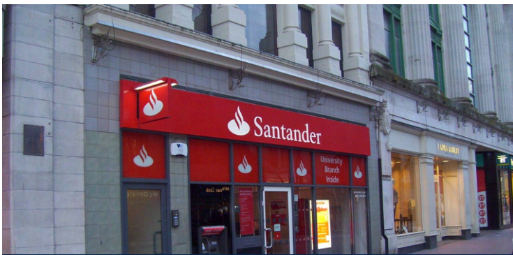
Basement damp proofing at Santander Bank, Marylebone
