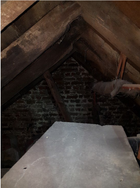
Left: The rafters to the rear roof slope.
