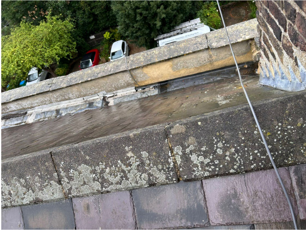
Above: An image that was taken prior to the scaffold being erected. This shows the dilapidated front lead gutter behind the parapet.
