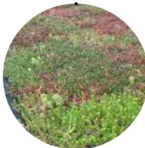
New green roof covering with pebble border
