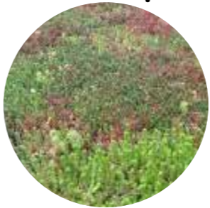
New green roof covering with pebble border
