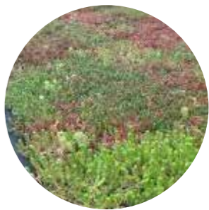
New green roof covering with pebble border
