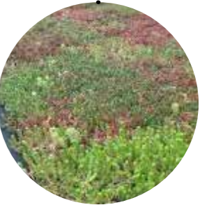
New green roof covering with pebble border
