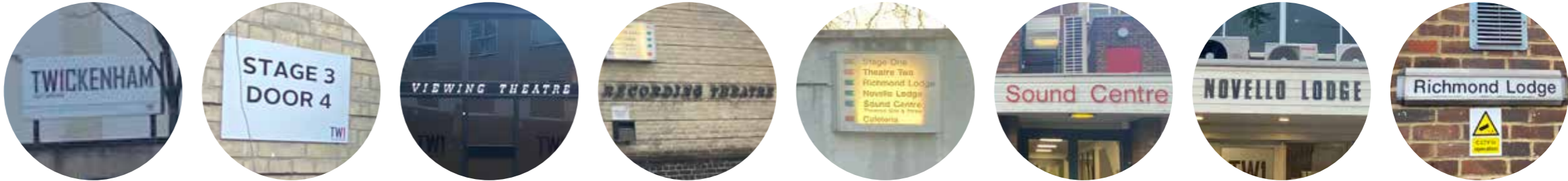
EXISTING SIGNAGE/FACADE CONDITIONS
