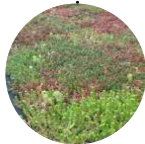
New green roof covering with pebble border
