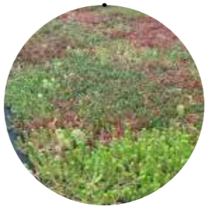
New green roof covering with pebble border
