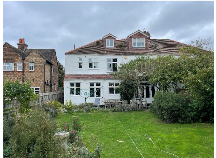
Figure 3: Rear elevation from the garden showing the adjoining neighbour's roof (No. 9) and No. 5 Nylands Av.
