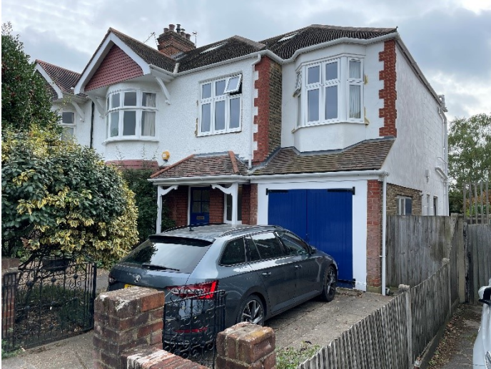
Figure 2: Front elevation facing Nylands Avenue showing the adjoining building to the left (No. 9 Nylands Avenue)
