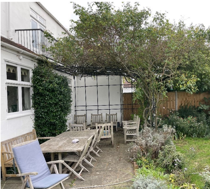
Figure 4: Garden patio view and No. 9 Ground floor rear extension's flank wall
