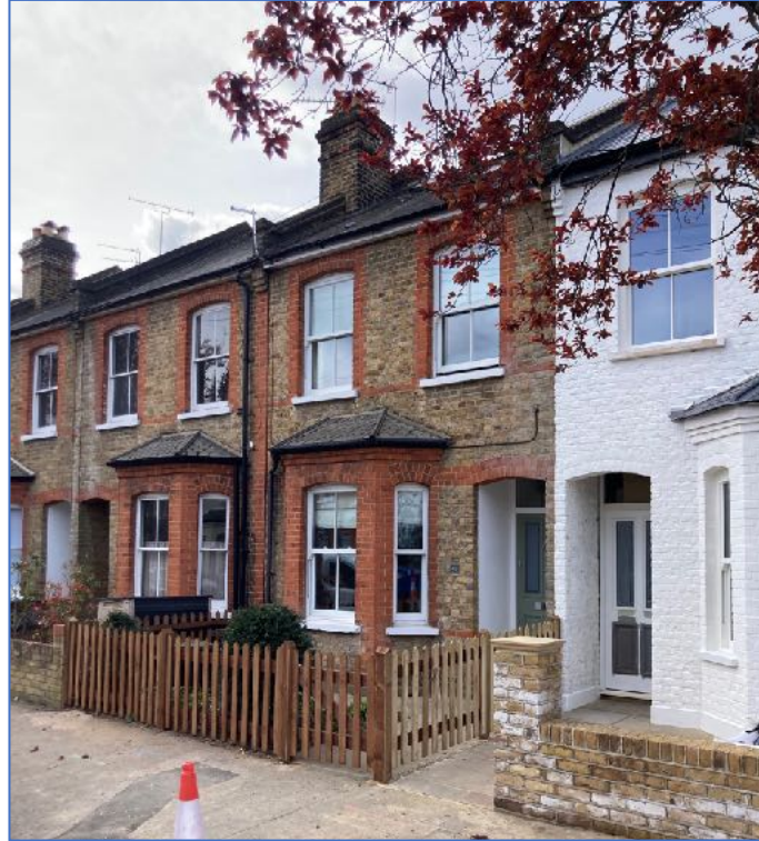
Existing street view of N°41 Arlington Road.
