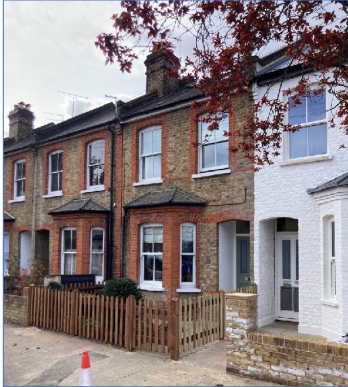
Existing street view of N°41 Arlington Road.
